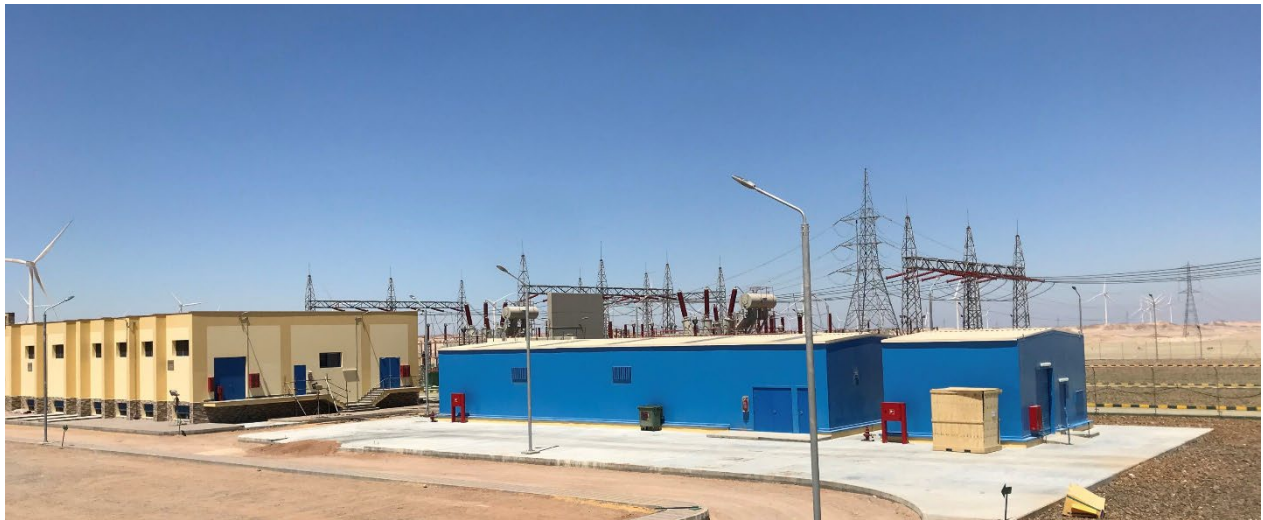
Control building, LTSA building and warehouse
