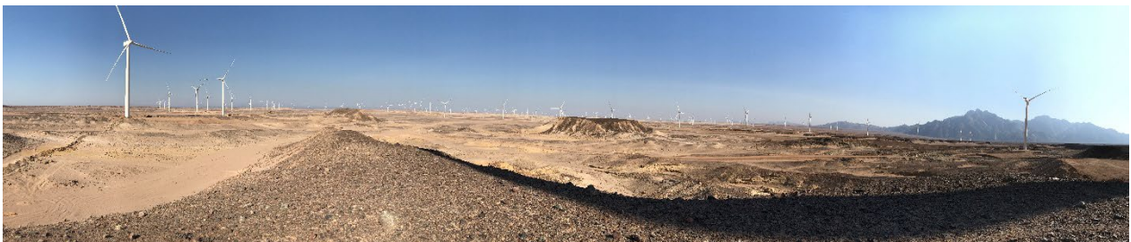
The 125 wind turbines of the farm are installed
