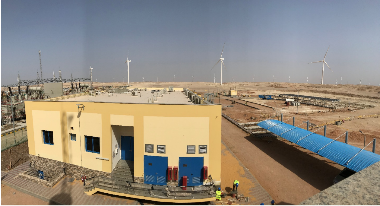
Control building, parking shed and chemical warehouse under construction
