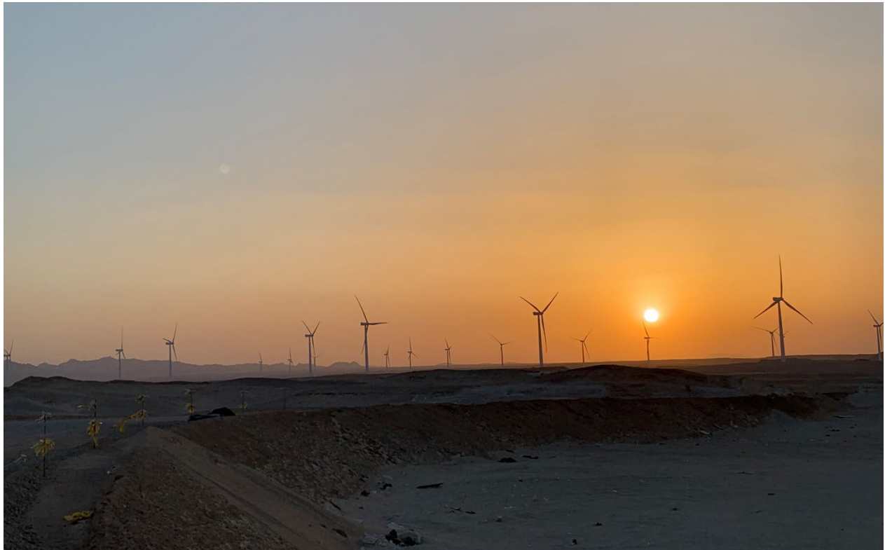
More than 50% of the wind farm turbines are operational
