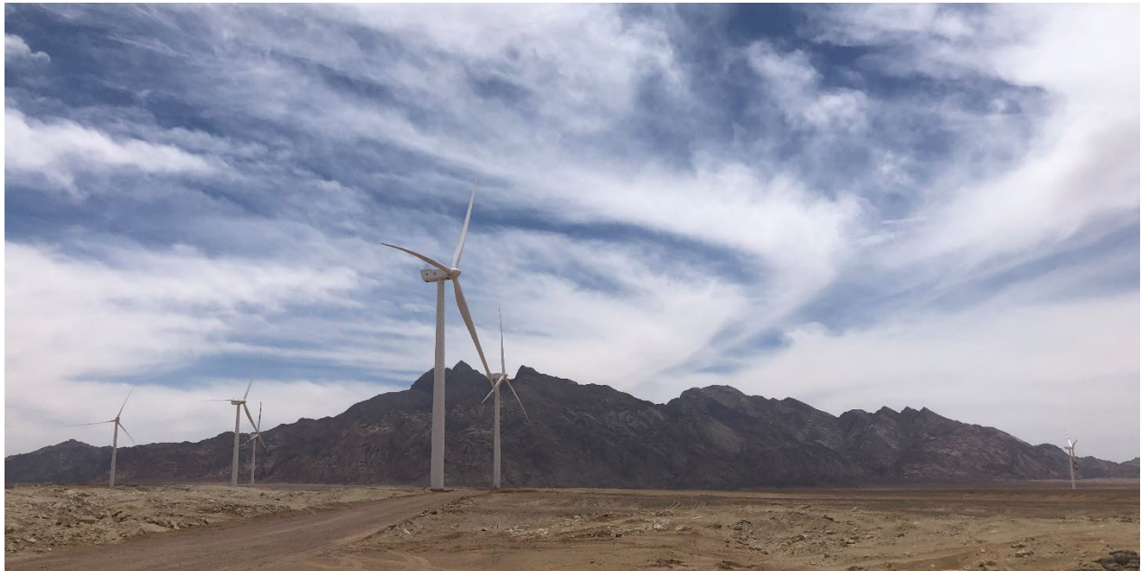
First wind turbines being commissioned and energized
